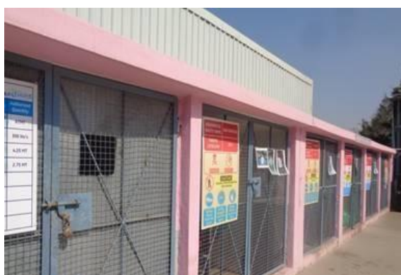
Fig 1. Hazardous Waste Storage Unit
